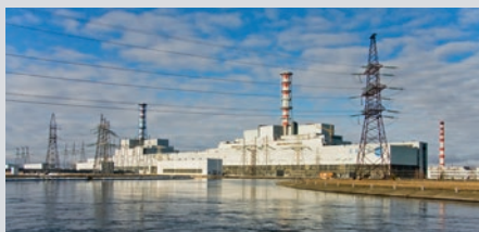
Branch Office of Rosenergoatom Joint-Stock Company – Smolensk Nuclear Power Plant
